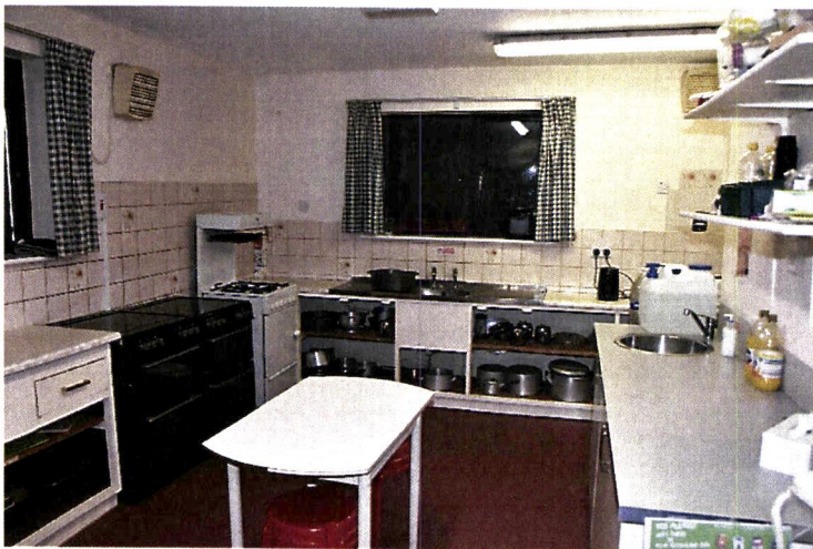
Item 2 Works (internal): Kitchen facilities to be renewed.
