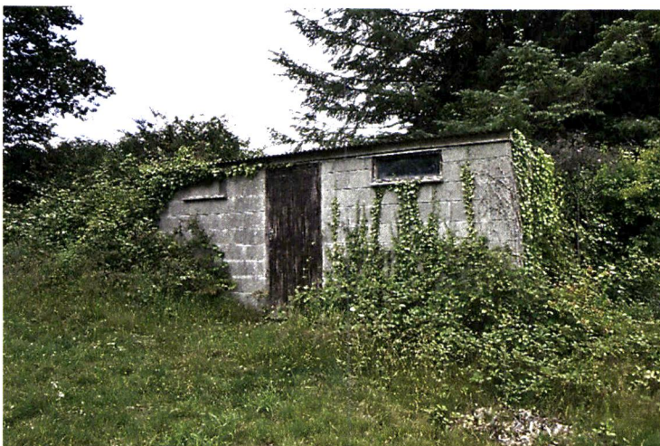
Item 4 Works (Shed): Improvement works to existing shed.
