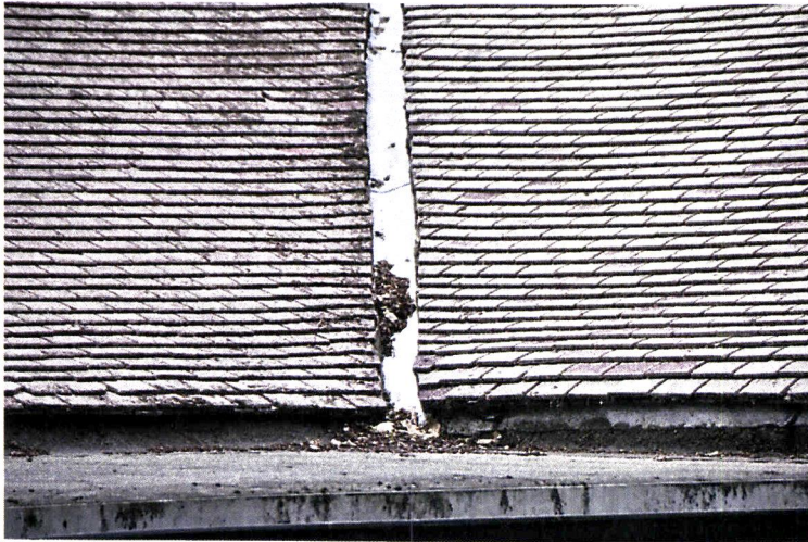
Item 1 Works Clear vegetation and repair flat roof section.
