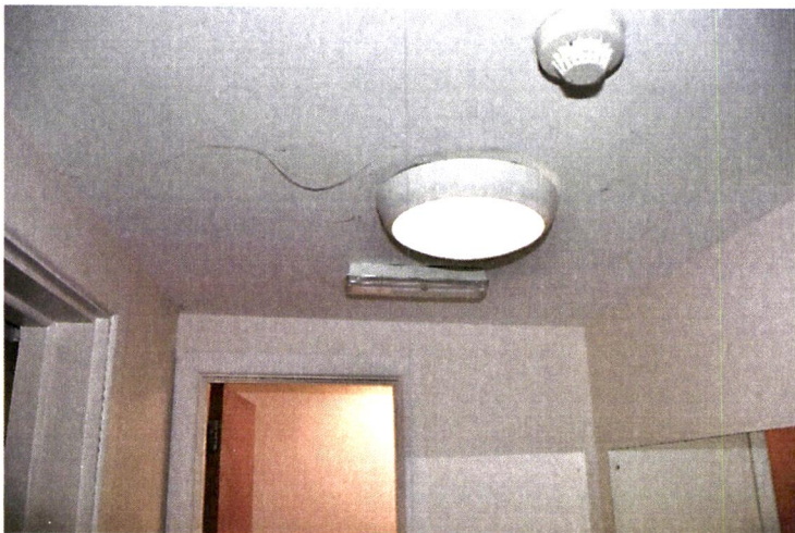
Item 2 Works (internal): Installation of mechanical extract ventilation to WC space.
