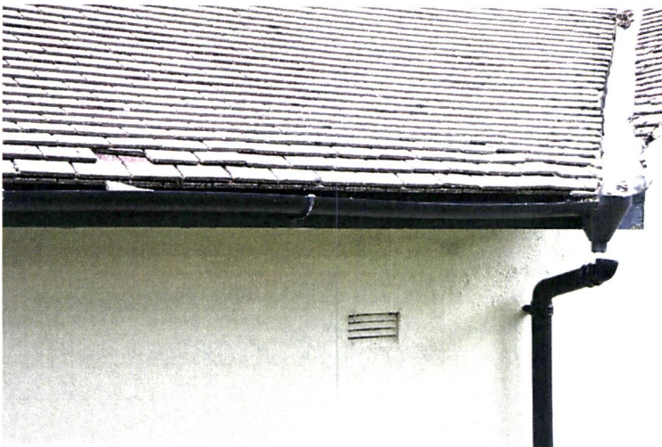
Item 1 Works: Replace slates and repair guttering and connections.
