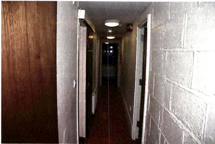
Item 2 Works (internal): Replacement of fire doors to two dormitories.
